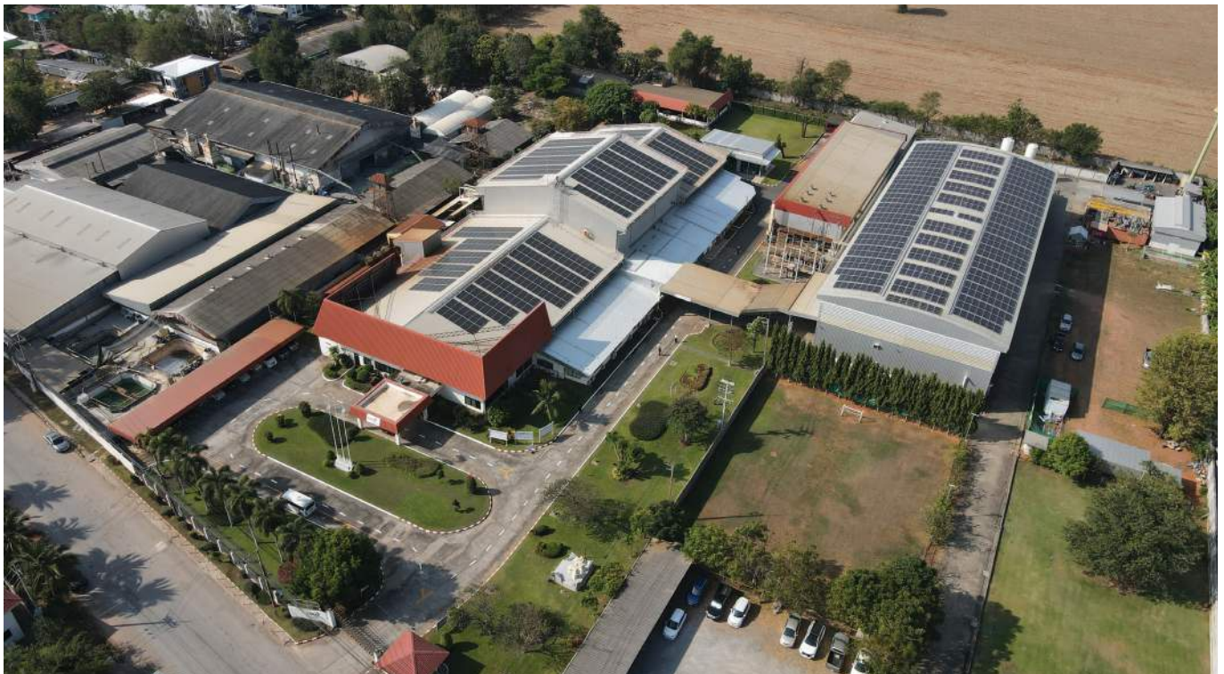
Two solar rooftop projects: left (2022), right (2021)
