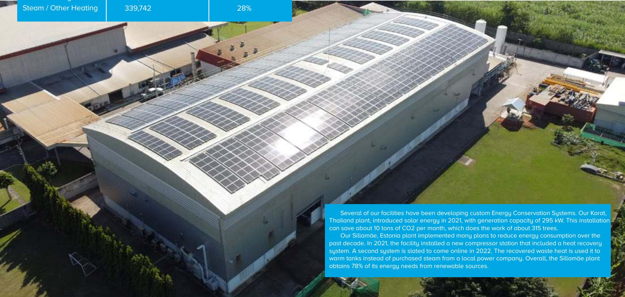
Several of our facilities have been developing custom Energy Conservation Systems. Our Korat, Thailand plant, introduced solar energy in 2021, with generation capacity of 295 kW. This installation can save about 10 tons of CO2 per month, which does the work of about 315 trees.
